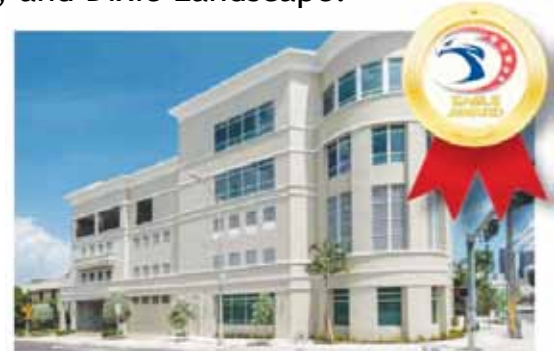
Miami Lighthouse Academy Expansion by Miller Construction: 2022 Eagle Award for Excellence in Construction
